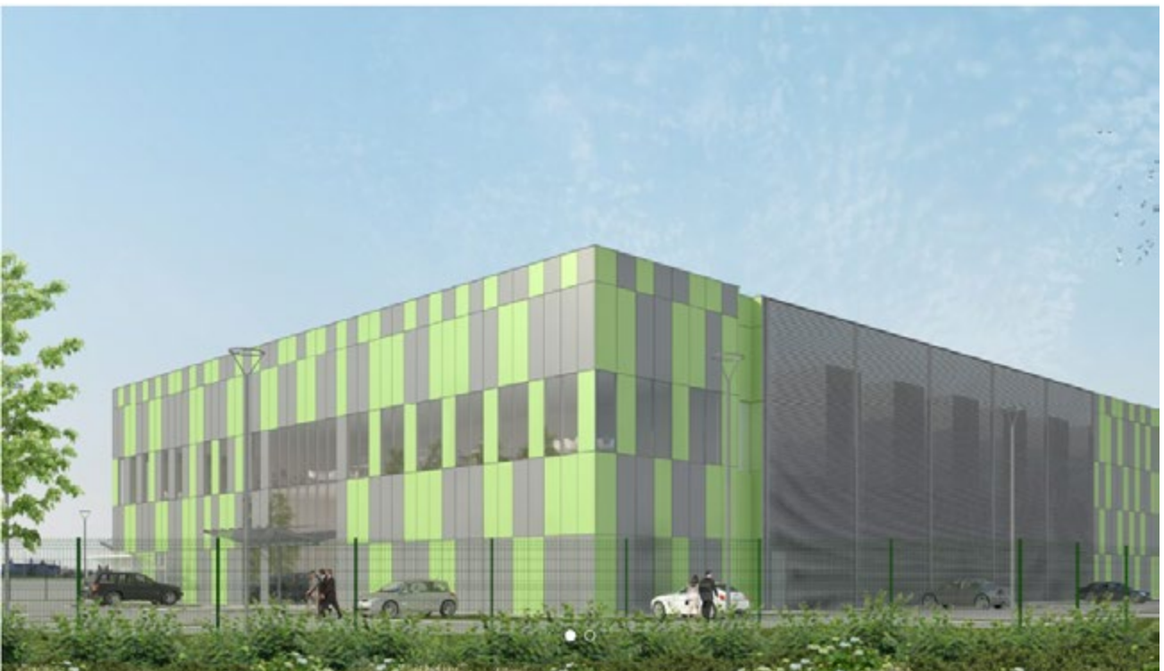
Data center Virid iData, Ferrières-en-Brie (77)/ ©R-b Architectes
