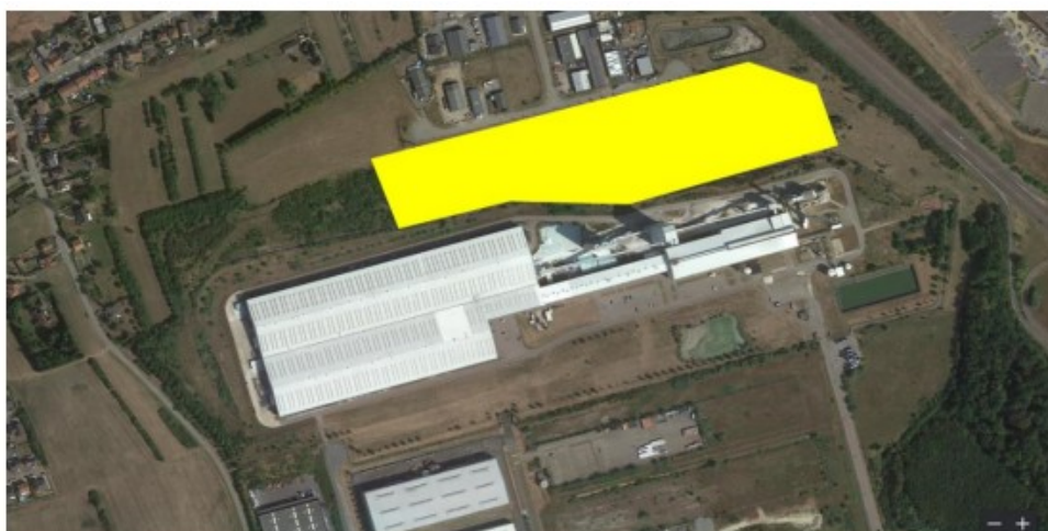
Figure 6: Localisation du champ photovoltaïque PV2
